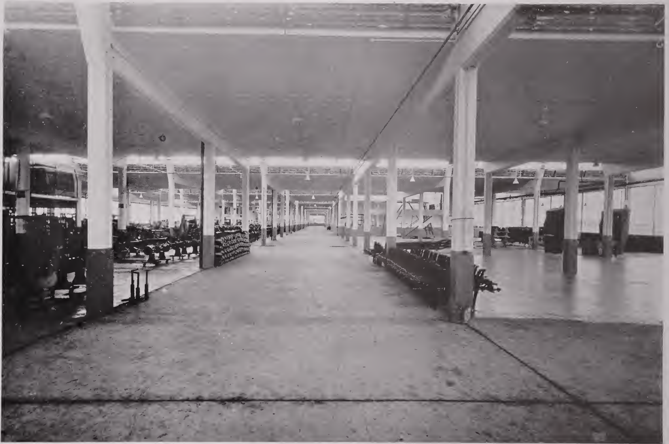
LOOKING DOWN MAIN AISLE FACTORY BUILDING NUMBER TWO
